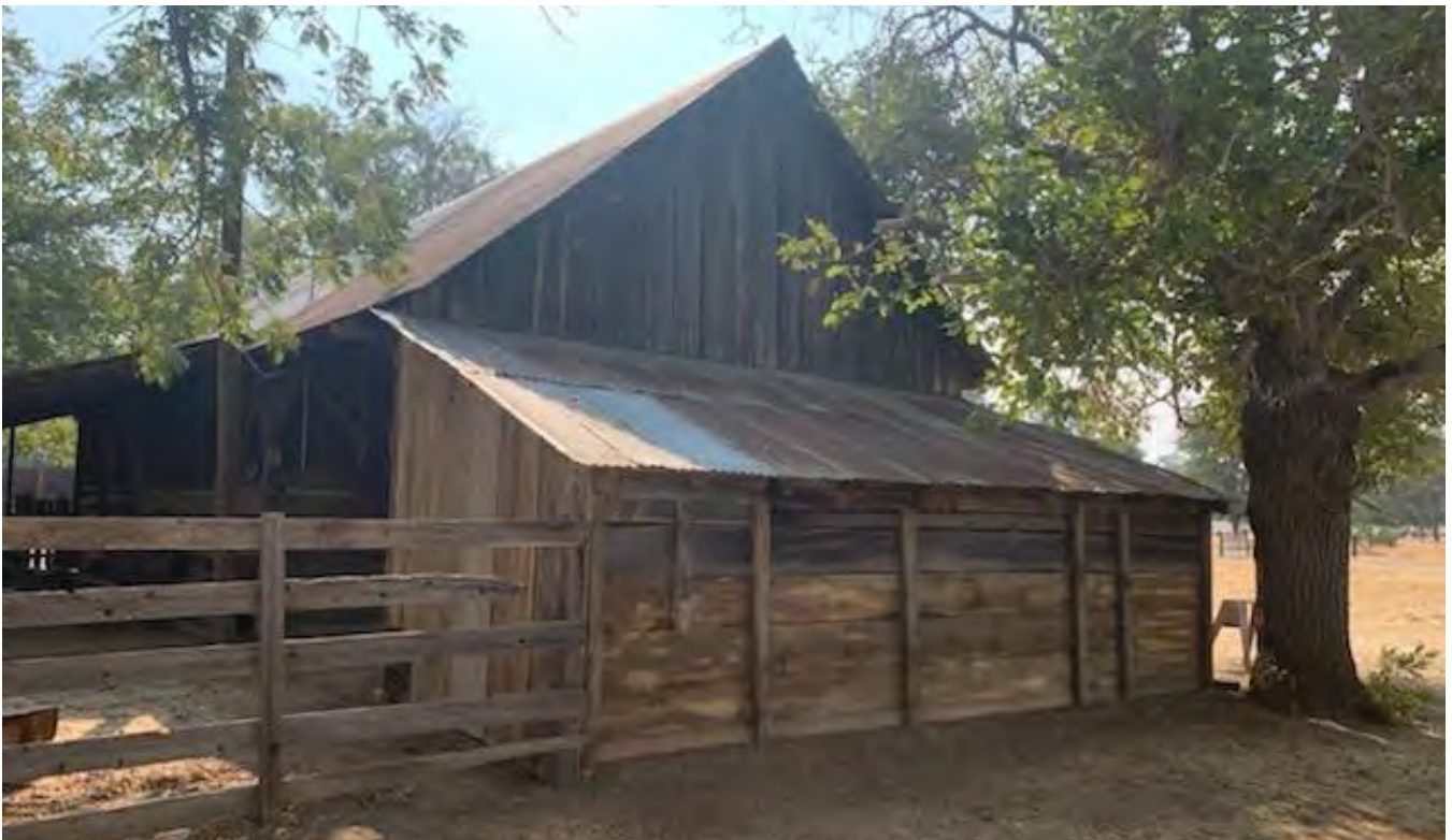
Repairs, including new foundation work, have stabilized the shed, keeping it from collapse.
